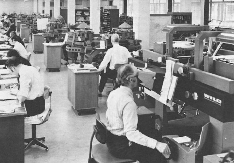
Above: the plotting room at Ordnance Survey in the 1970s. In the foreground an operator is working at a Wild A10 Autograph.
