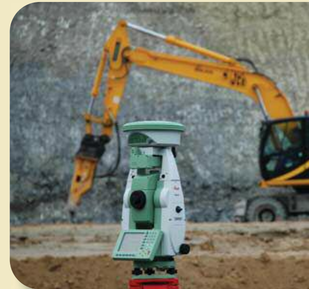
Below: a Leica System 1200 Smart Station with GPS on a highways project.
