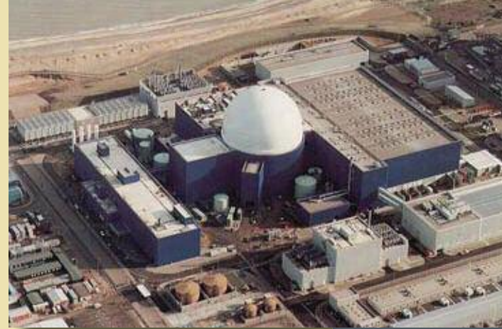
Above: Sizewell B nuclear power station.
